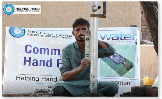
Community hand pumps are perfect for villages with common underground water sources, providing an affordable and simple solution for families with limited resources. These suction hand pumps, made of durable cast iron, are easy to install, maintain, and repair at the village level without specialized parts. Each unit consists of two local hand pumps to serve the community's water needs efficiently.
